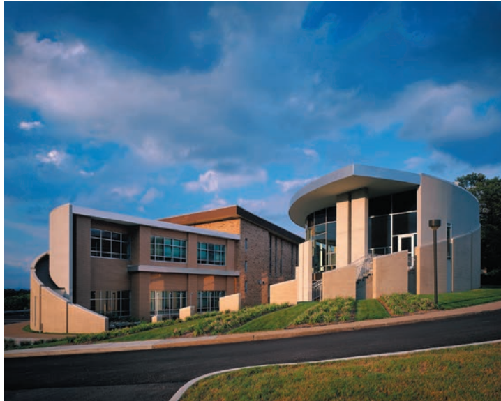
Brick site walls
