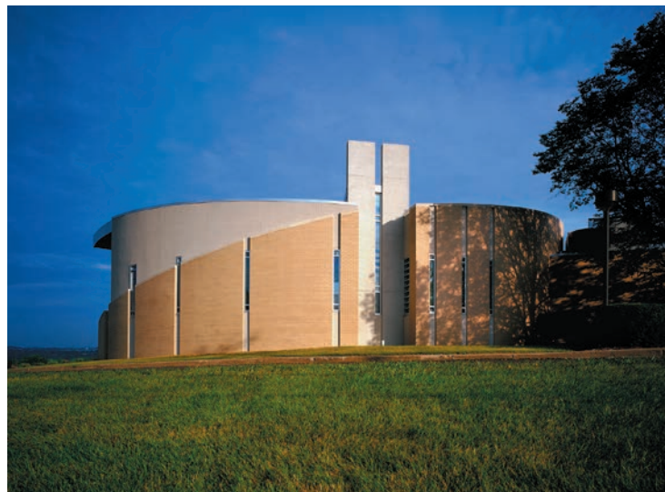
Eastern wall, morning light
